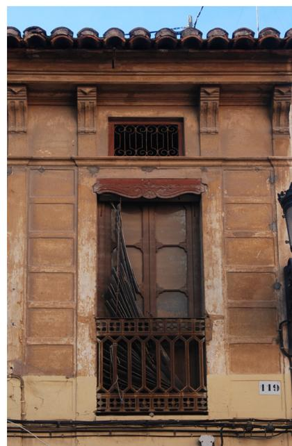
Figura 209. Guardamalleta de madera(1900) calle Barraca 259. (Pastor, R. 2011)
